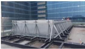
3. Pool panel positioned above checkered plate
