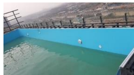
6. Equipments installed after liner fixing
