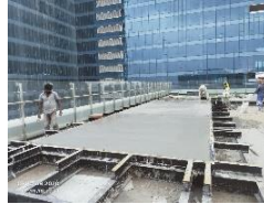
3. Pool panel positioned above checkered plate
