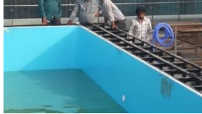
9. Frame for wooden panel finished
