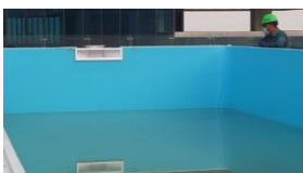
7. Skimmer fixed after liner fixing
