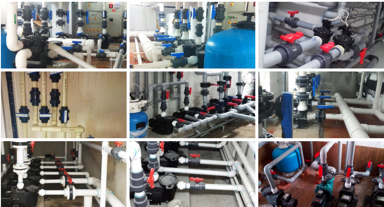
Photo courtesy: Aqvastar's specialist pool contractors installed in various part of India.
